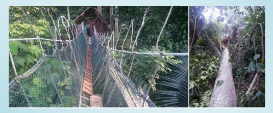
Damages to the FRIM Canopy Walkway caused by the recent storms. A Melembu tree fell onto the second part of the walkway, causing stress on the whole system.
